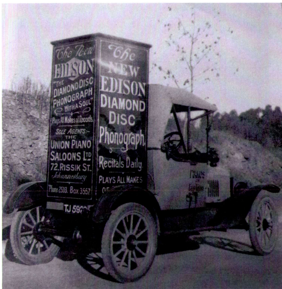
From Walter Norris' albums comes this photo of a novel South African advertisement for the Edison Disc Phonograph. The Ford Model T appears to have two electrical cables running from the driver's compartment to the rear of the car. Could these be for illuminating the display?
